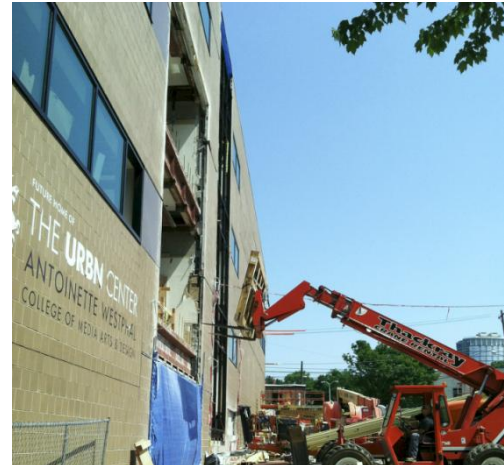
Figure 2: East curtain wall installation. (Photo Property of Drexel University)
